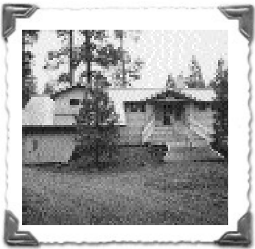
The front entry to the Mack house at Black Butte Ranch.
